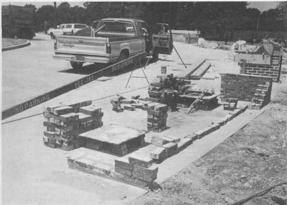
ALL THAT'S LEFT: Most of the 10,000 bricks salvaged from the Old Administration Building are being used to face planters and walls in the Commons area. The bricks were saved after several student groups protested the building's demolition early last summer [photo by Dan Swanger].
